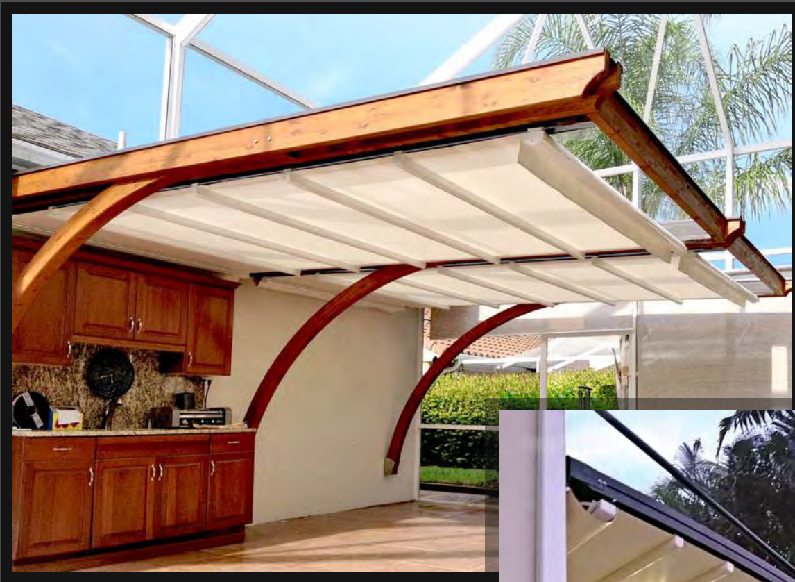
Cantilevered roof with contoured ▲ support arms
